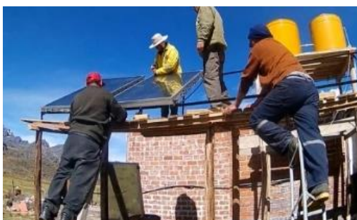
Fig. 12: Installation of the water heater (2 tanks of 300 liters, 5 solar collectors)
