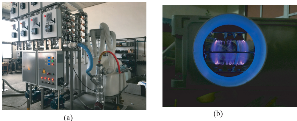
Figure 2. Installation for the intensive ozonization of landfill water (a); and the process of ozone synthesis in a glow discharge (b).
