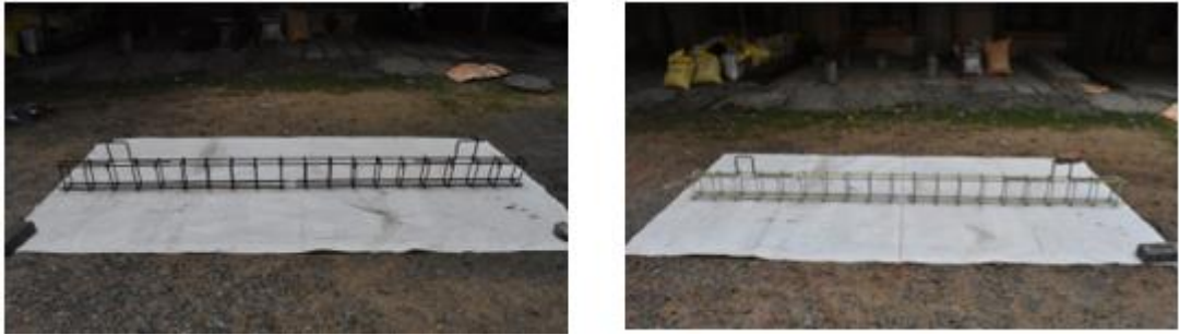
Figure:2 Reinforcement structure of beams
