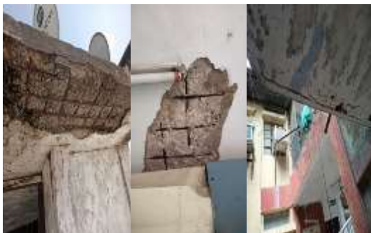
Fig. 10 Grouting and re-casting or plastering of (existing) damaged ceiling plaster
