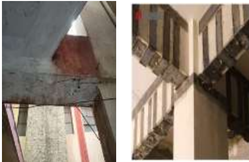
Fig. 9 External plate bonding for column and beam repair
