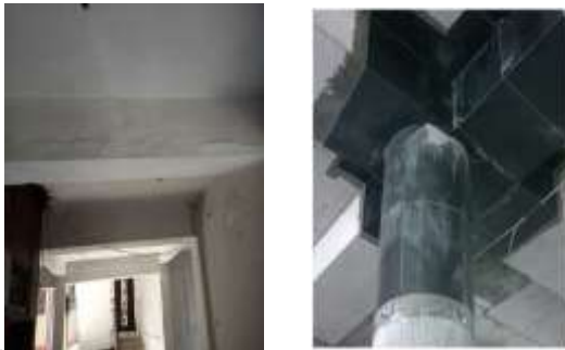
Fig. 7 FRP for retrofitting of building
