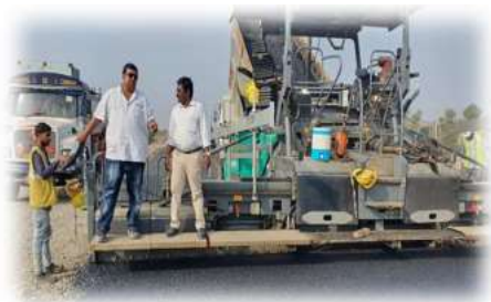
Fig 4 : Laying of Road using Modified Bitumen.
