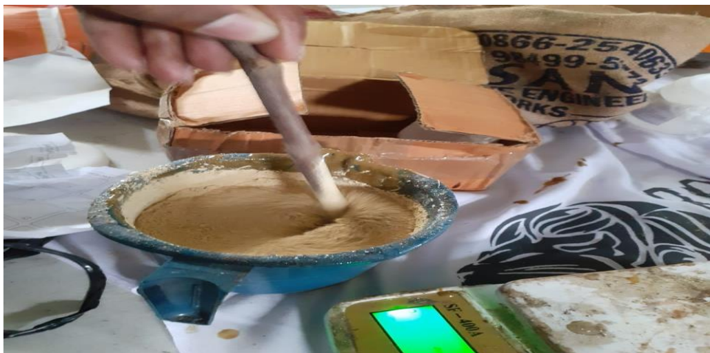
Fig: Mixing of materials
