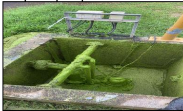
Figure 8: Condition of Submersible Pump that Needs to be Maintained
