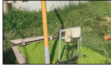
Figure 7: Condition of Overflowing Sewage Tanks
