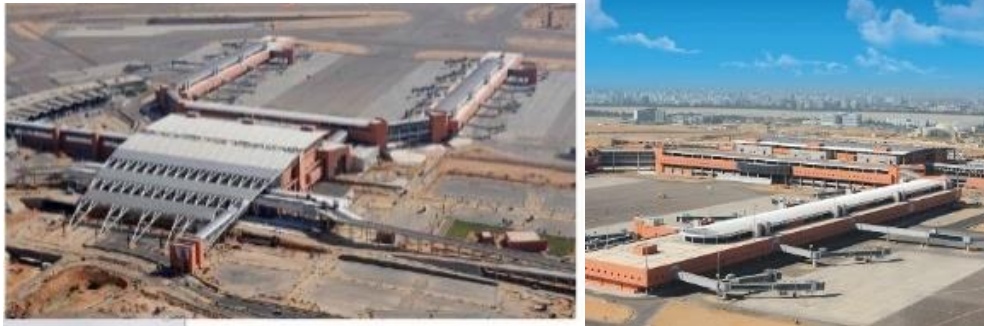
Figure 2 Cairo International Airport – Terminal-3 (google image.com)
