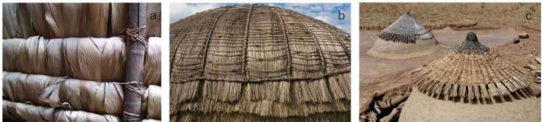
Figure 5 Examples of Vernacular Architecture Utilizing left overs of local Agriculture in Construction (a: palm and vine weaved roof, Ecuador - b: dried grass and stack beehive structure, South Africa - c: stack and straw roof, Ghana (source: Habitat: Vernacular Architecture for a Changing Planet, Piesik, 2017)
