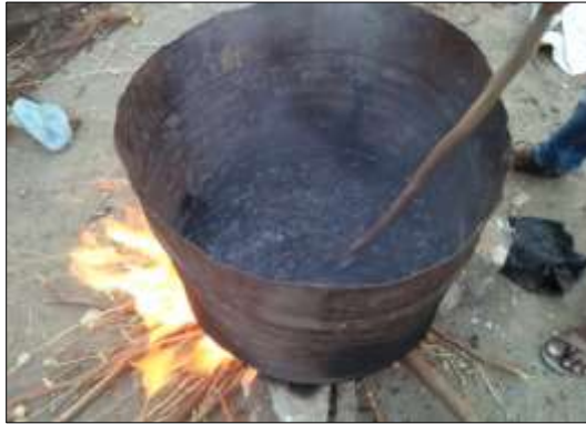
Figure 2. Melting and mixing of plastic waste bricks
