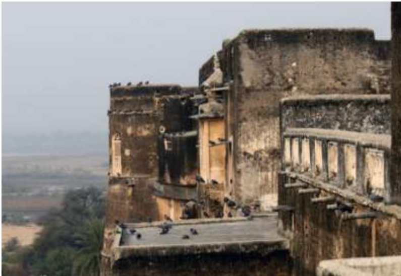
Figure 2: Meja Fort Rajasthan ((Source: The Better India)
