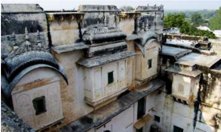
Figure 3: Meja Fort Rajasthan (Source: The Better India)
